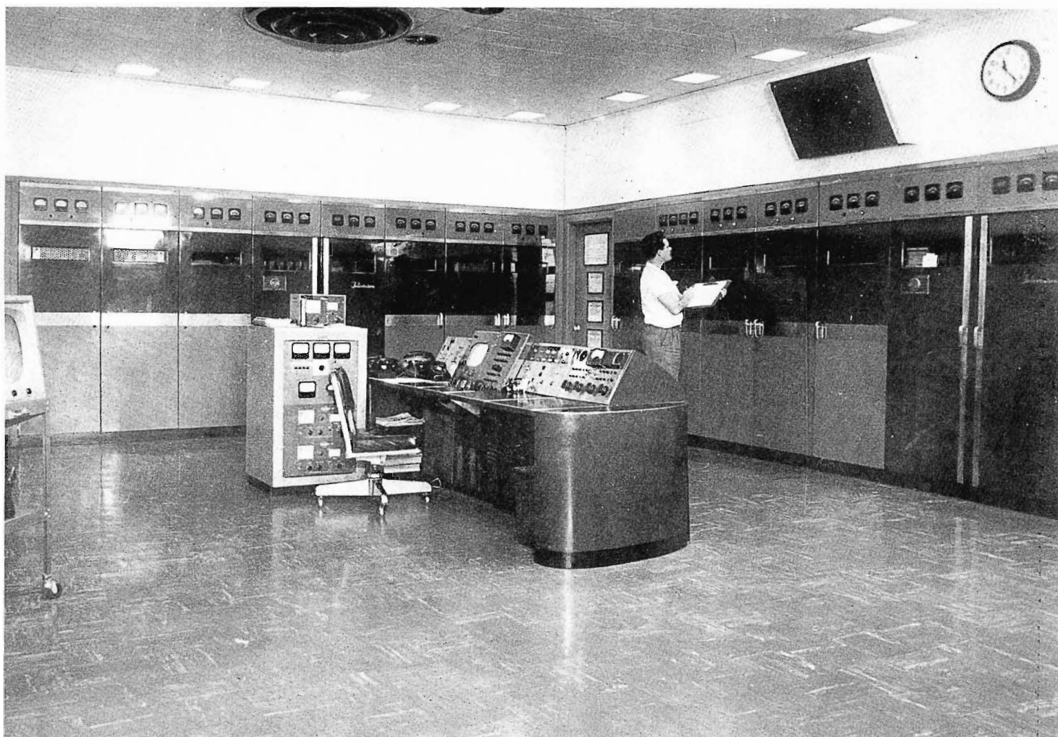
The two new 30 kW TT-30FL transmitters occupy less floor space than the TT-25 and TT-5 which they replaced. This "bonus" space in the photo above is being refurbished and will be occupied by the video tape operation which is scheduled to move from typically cramped quarters next to Master Control.
